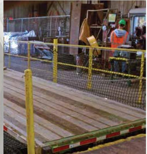
Fall protection measures using safety nets are considered necessary when alternative means of fall prevention are not feasible.
